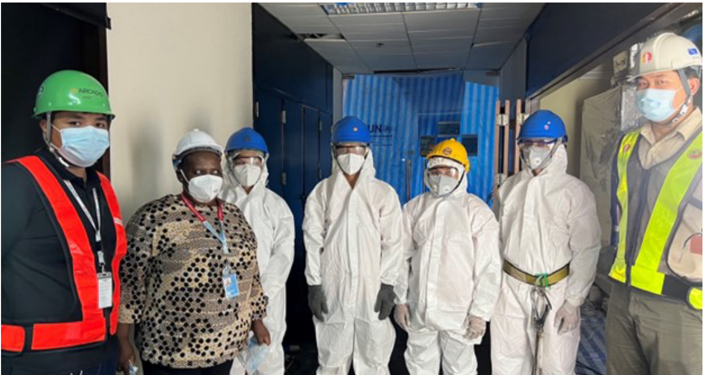
OSH briefing for workers before hazardous materials removal
