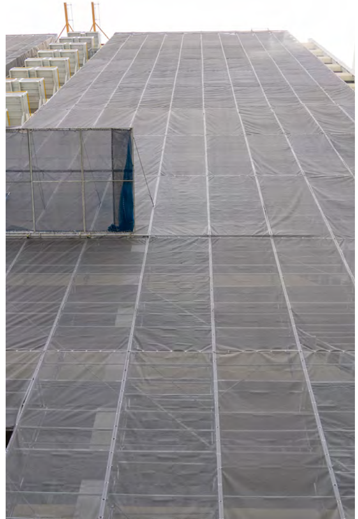
Scaffolding Installation for Phase 1 Construction
