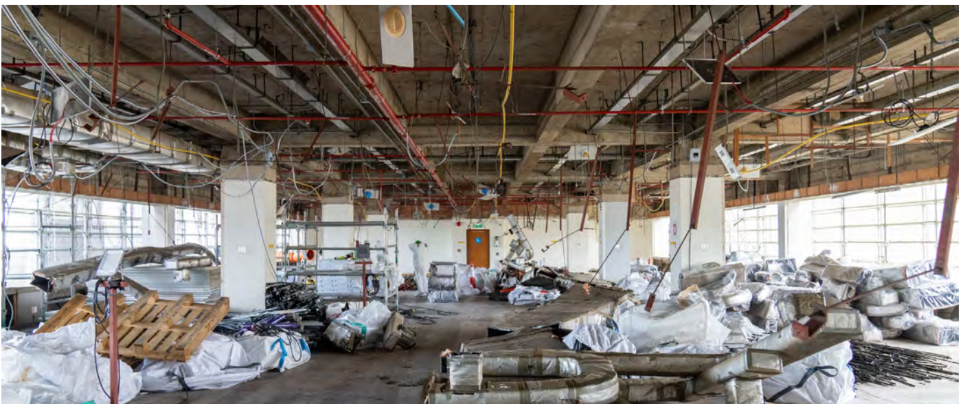
Interior Demolition Works
