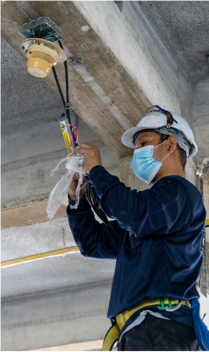
Interior Demolition Works - Existing Smoke Detector Removal
