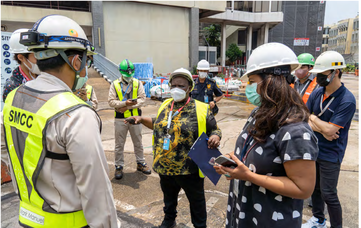
Safety and Health Matters: Susan conducting random safety inspections at the construction site
